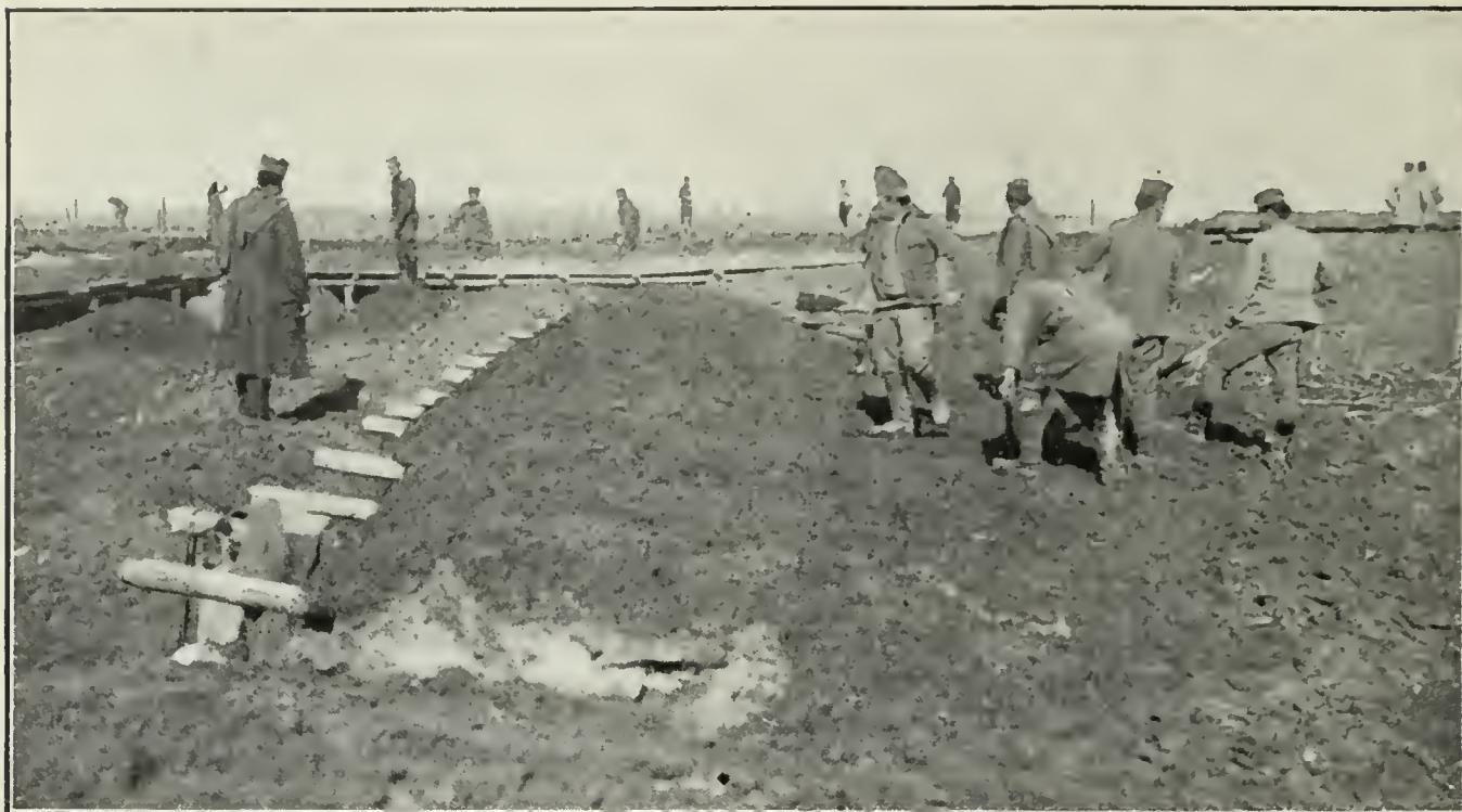
SERBIAN SOLDIERS COMPLETING TRENCHES AND PUTTING WIRE ENTANGLEMENTS AROUND THE FORTS OF BELGRADE.
