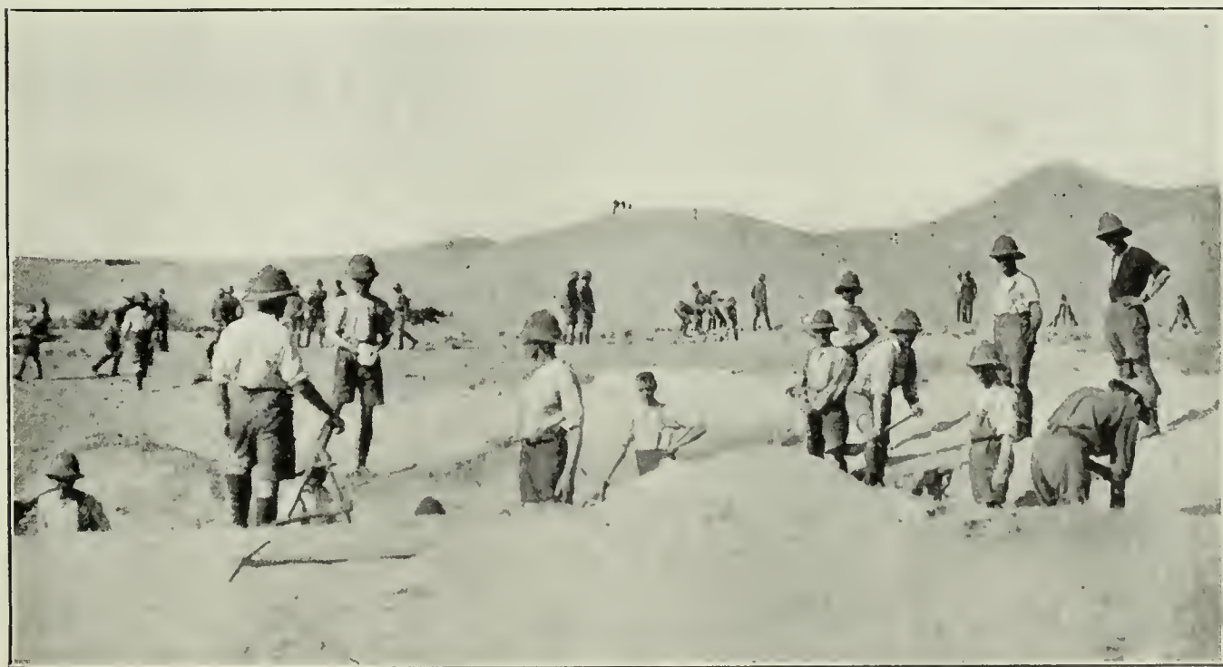
BRITISH SOLDIERS DIGGING TRENCHES IN THE DESERT.
