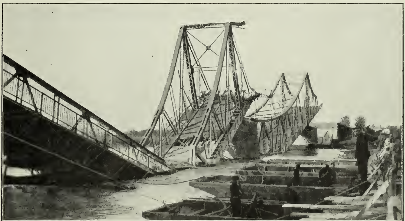
BRIDGE OVER THE DNIESTER DESTROYED BY THE AUSTRIANS DURING THEIR RETREAT.
