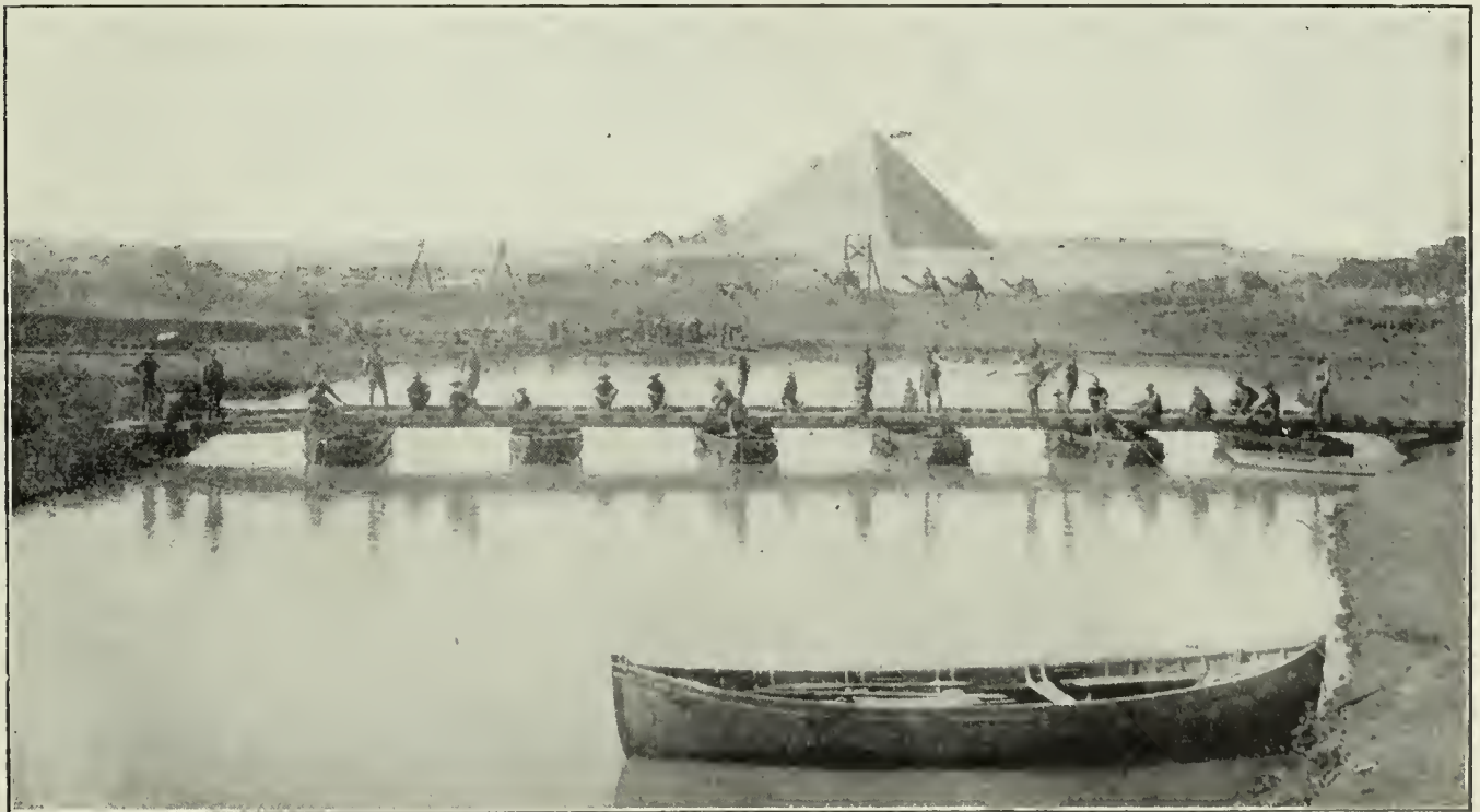
AUSTRALIAN ENGINEERS BUILDING PONTOON.
