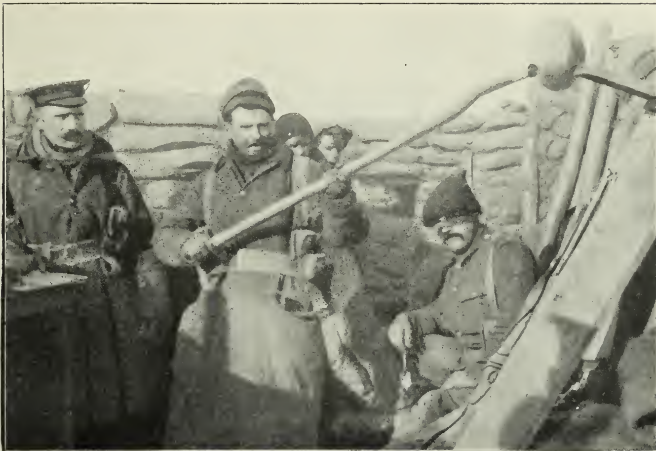
LADLING MUD OUT OF THE TRENCHES.
