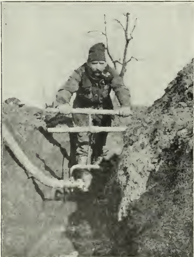
BRITISH SOLDIER PUMPING OUT WATER FROM A TRENCH.
