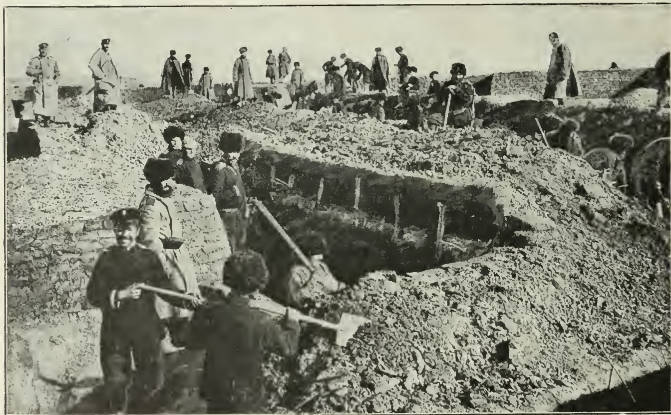
RUSSIANS DIGGING TRENCHES.
