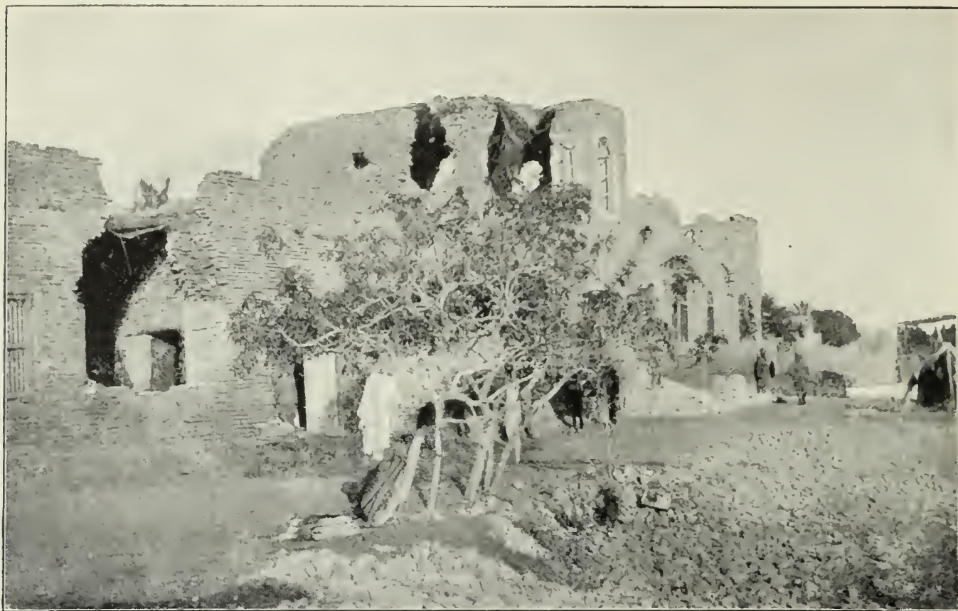
THE DAMAGED CUSTOMS HOUSE AT KURNA. How the Royal Navy left it.
