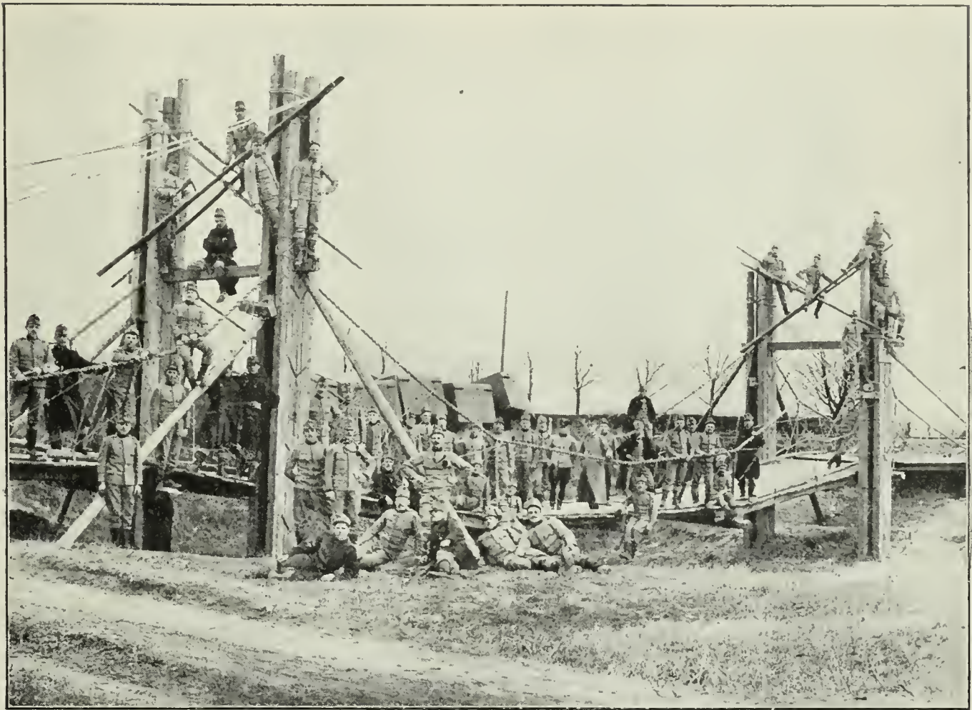
SUSPENSION BRIDGE CONSTRUCTED BY AUSTRIAN ENGINEERS.
