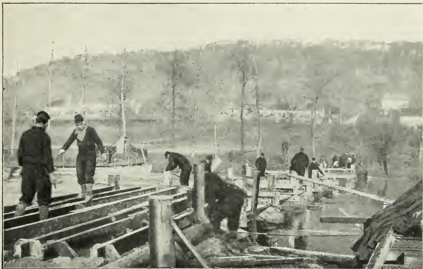
FRENCH ENGINEERS REPAIRING A BRIDGE.
